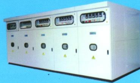
33kV VCB Five Panel
