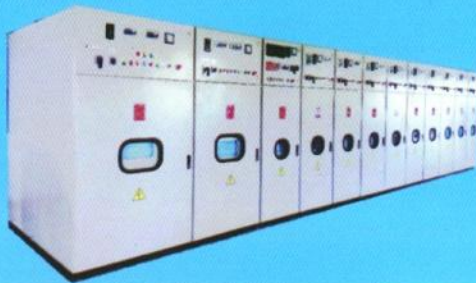
11kV VCB Line Up Panels
